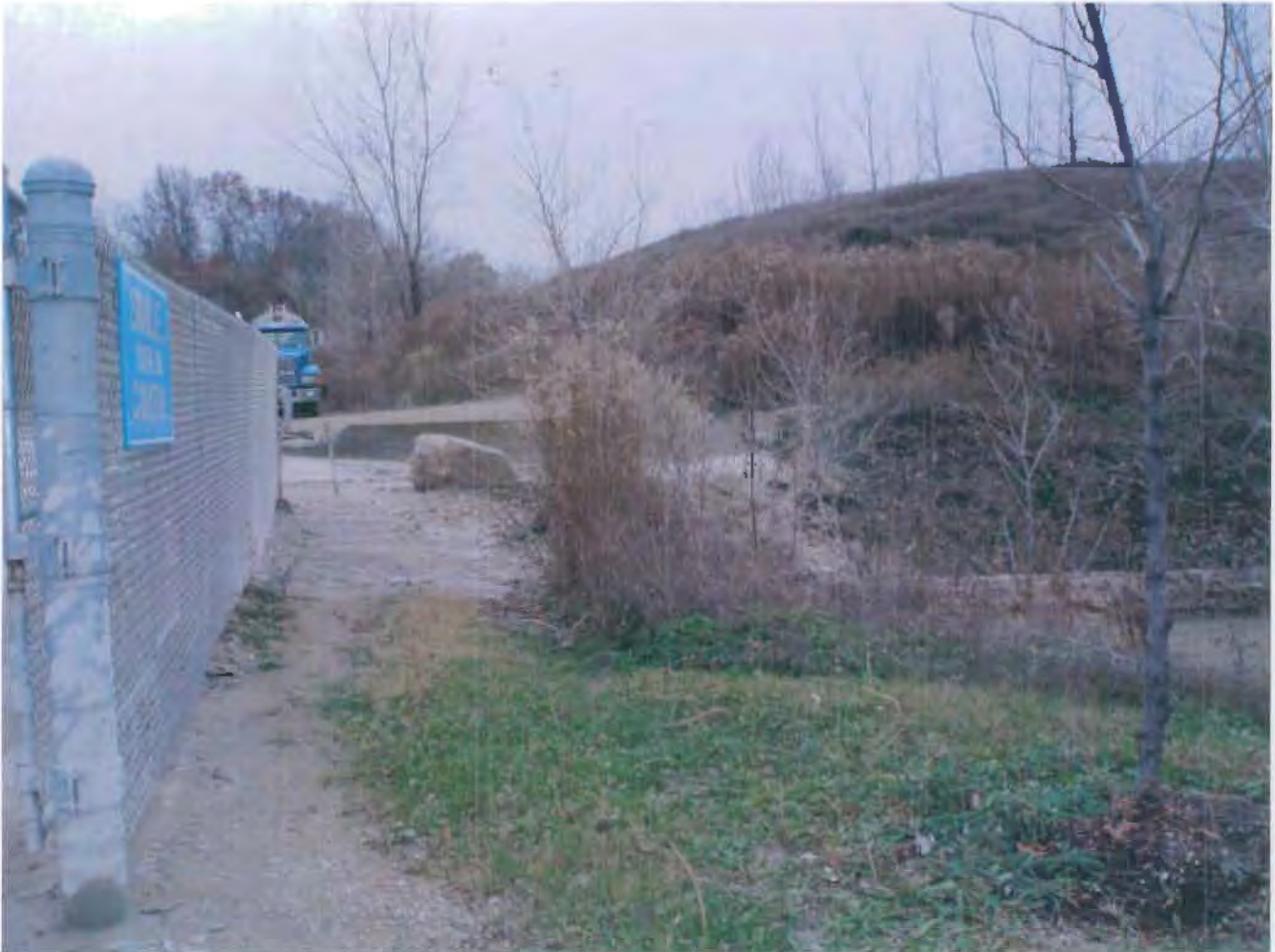
Photo 2 – shows how flow is able to run off the property from the wash area into the settling basin in the road ditch.
