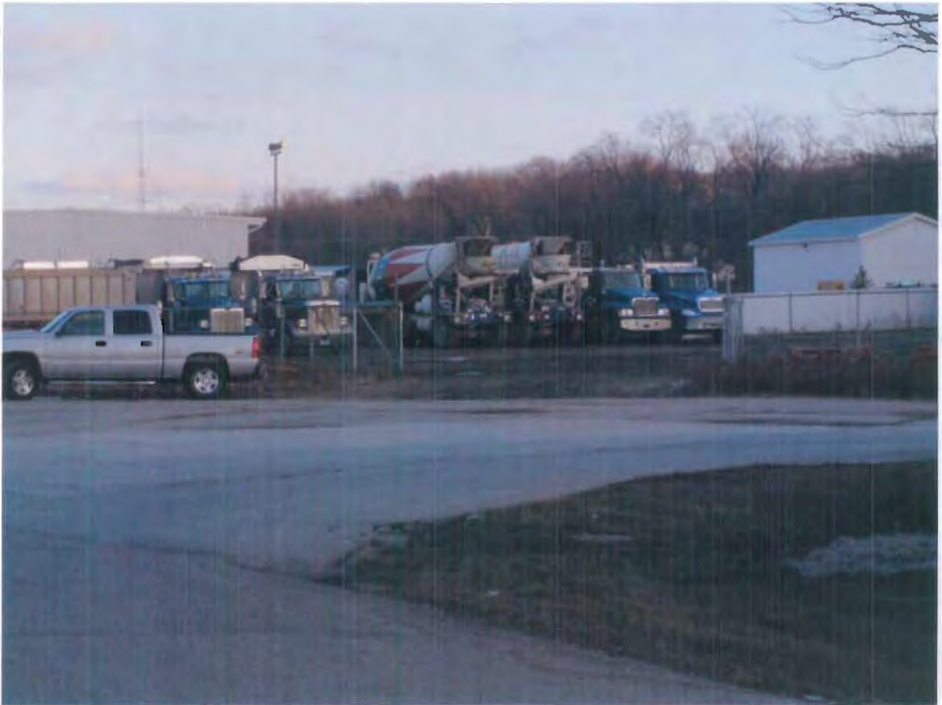
Photo 8 – Closer view of the unstabilized parking area. Note there is no paving or gravel in this area and there is some dirt being tracked on to the roadway.
