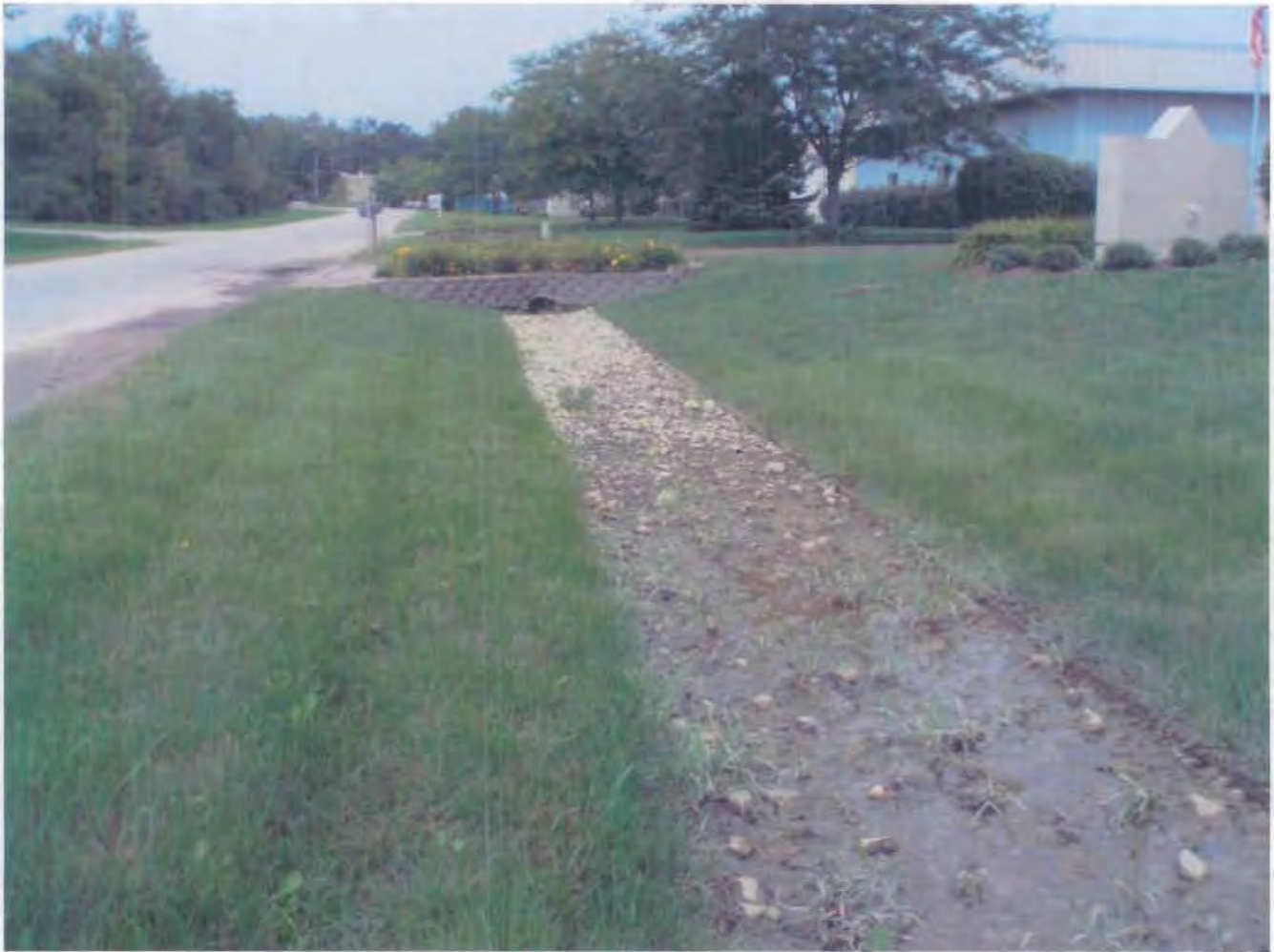
Photo 9 – A view of the storm ditch on the north side of Spring Ridge Drive, across from the facility.
