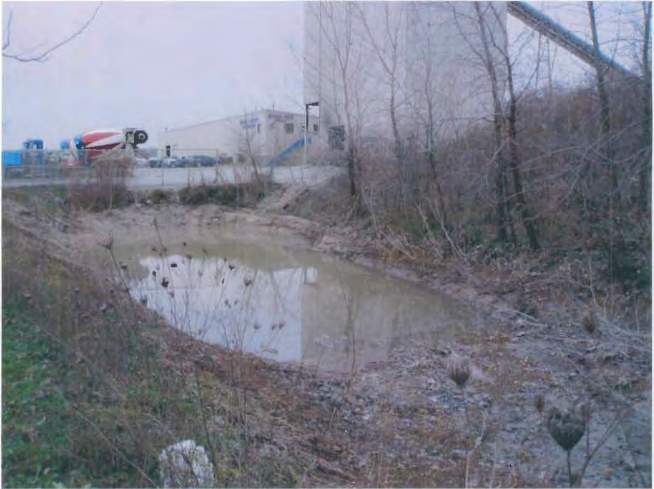
Photo 1 – Settling pond for concrete truck wash water adjacent to Spring Ridge Drive
