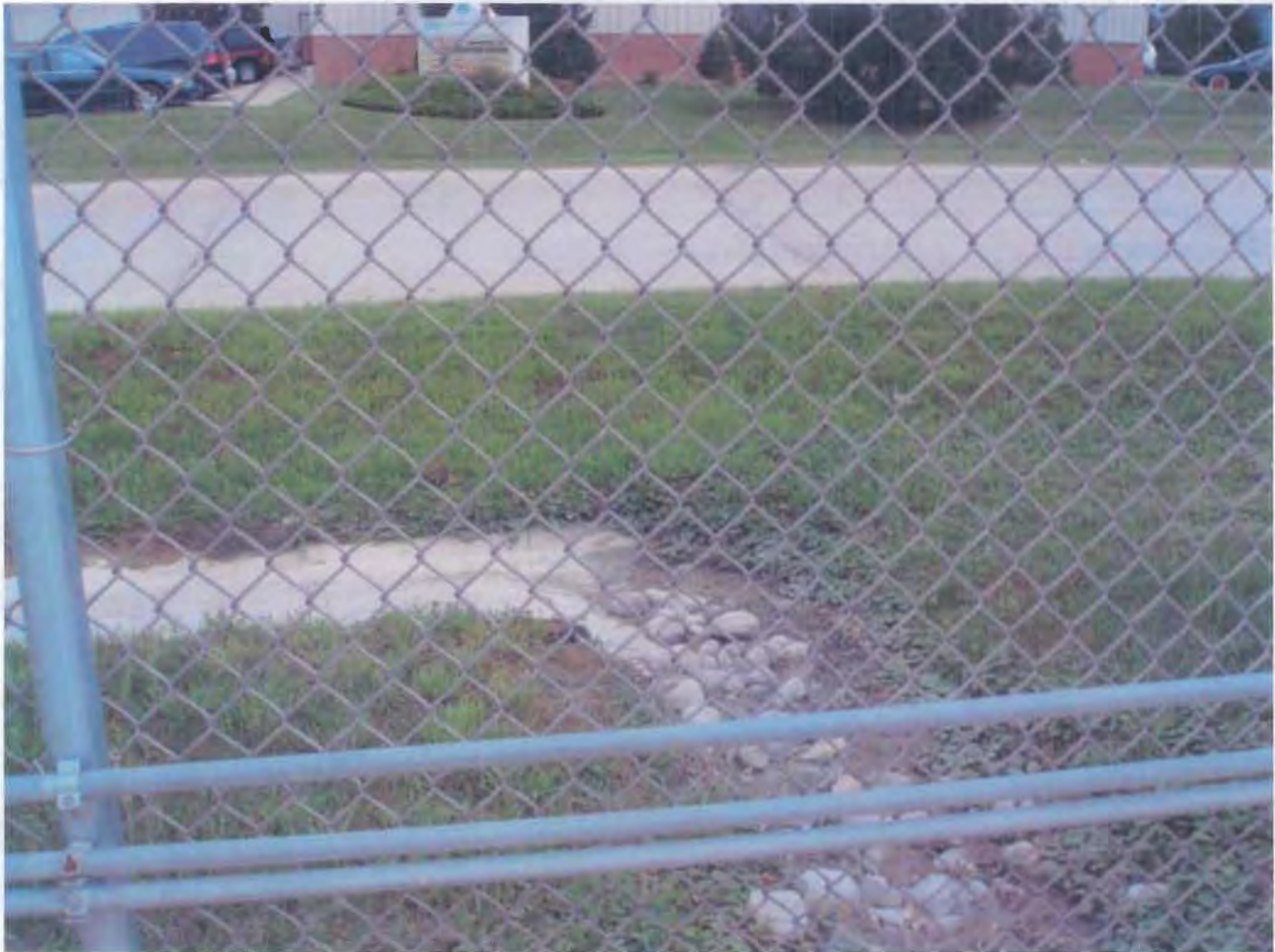
Photo 5 – This is where the discharge from the storm sewer in Photo 1 enters the road ditch. Note water quality and color in road ditch.
