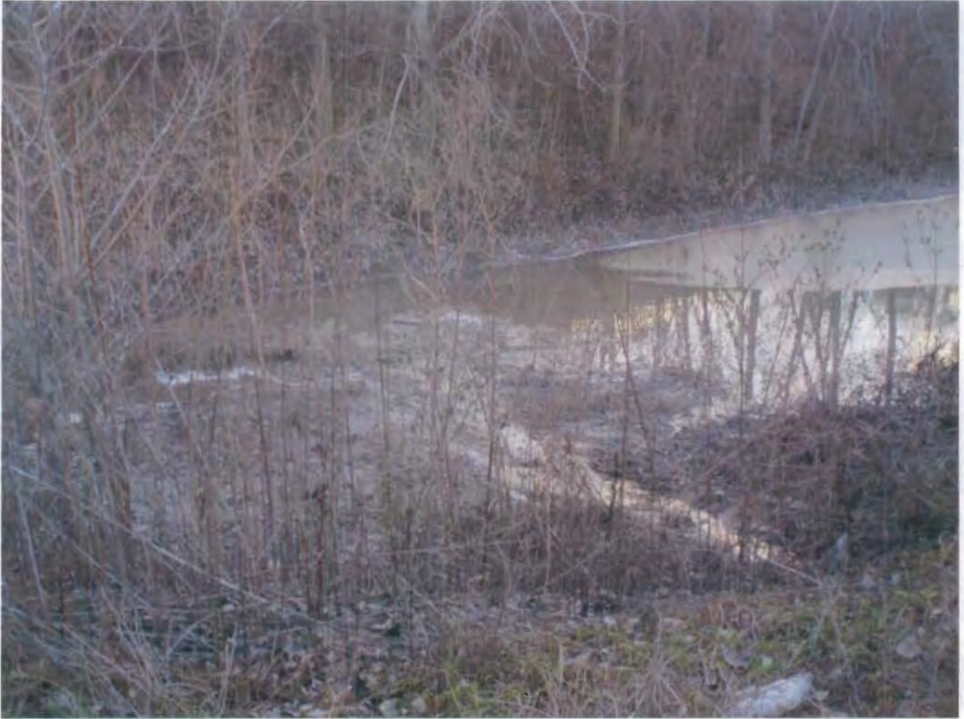
Photo 4 – View of settling pond west of driveway entrance, showing collected process material.
